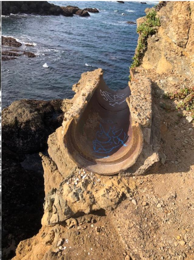
Photo 6: A section of drain near Glass Beach today showing coastal erosion and where waste water went.
